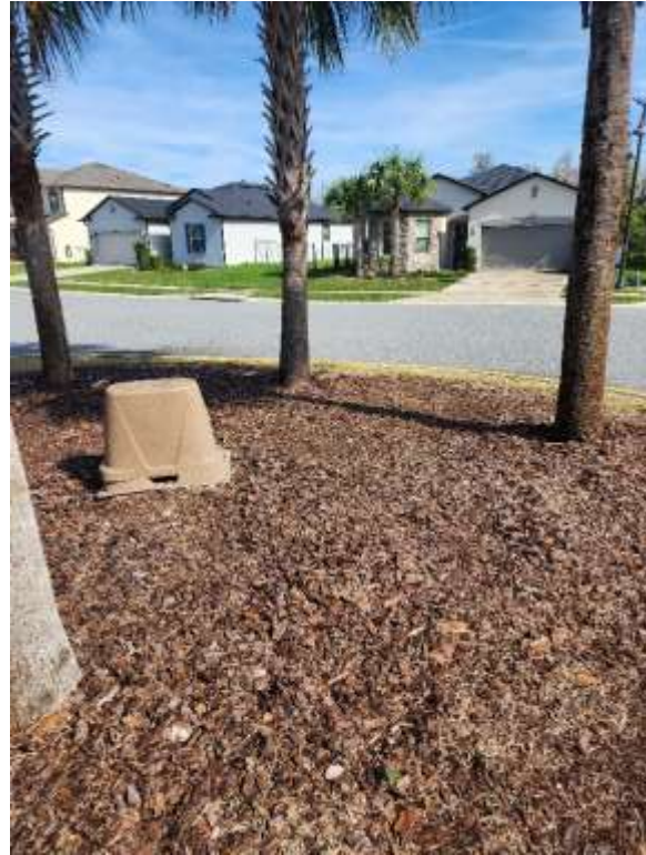
Butterfly Pea Island irrigation is now working.
